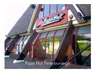
The unusual construction of the building has its roots in North American design with 6 huge timber 'A' frames providing the main structure for the building. The timbers which measure are 650mm x 180mm are made from 14 sections of soft wood laminated together to form the large sections of timber.
